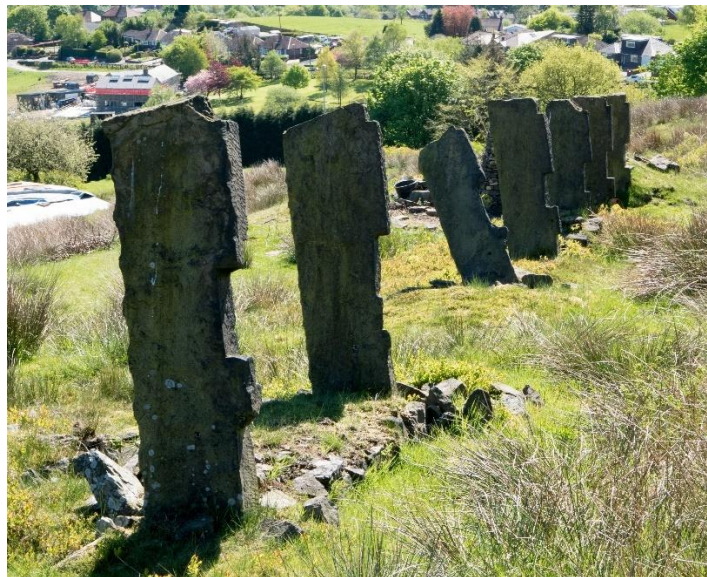
Figure 3. Remains of stone tenter-posts near Wall Hill, Dobcross, dated c. 1840. The notch at the top would hold the fixed upper bar of tenterhooks, the extended notch below housed the mobile lower tenterhook bar to stretch the cloth evenly.
