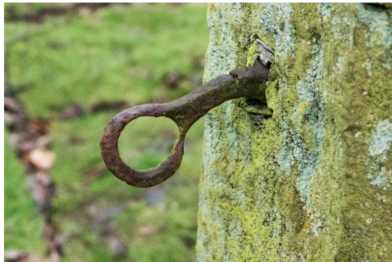
Figure 7. A closed loop about half-way down the side of the posts, aligned for rope to pass down the row.
